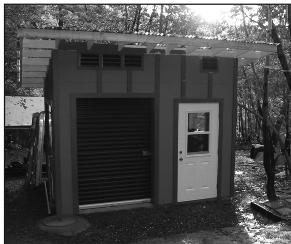
The new solar shed
