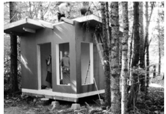
Kuti under construction
