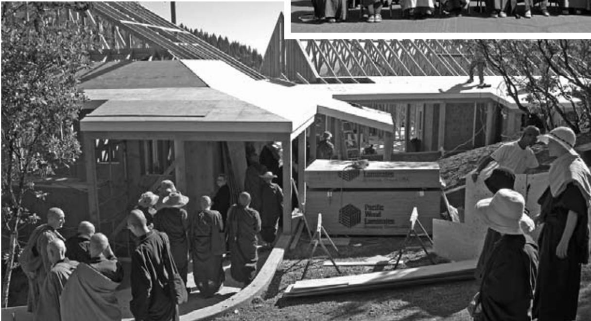
WMBG participants visit the new utility building at Abhayagiri
