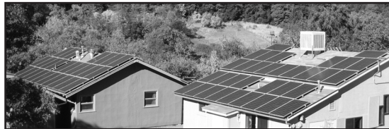
Cloister area solar array
